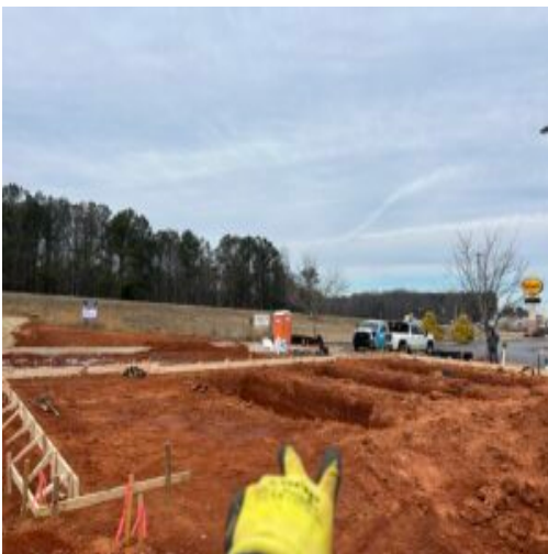
Looking from the southwest corner of building.
