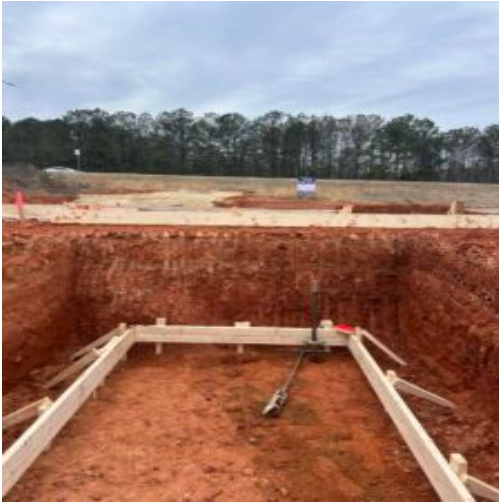
Another view of the lift pits.
