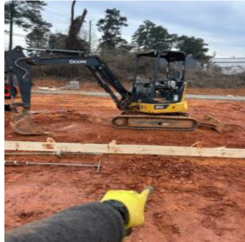
Contractor used excavator to scrape down 1.5 feet of hardened ground from the surface in order to perform hand auger/DCP test.
