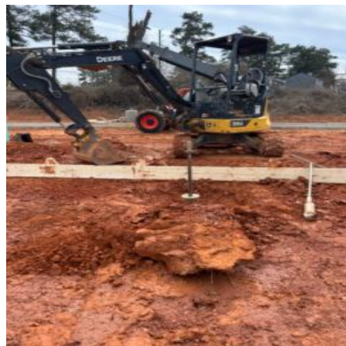
Contractor used excavator to scrape down 1.5 feet of hardened ground from the surface in order to perform hand auger/DCP test.
