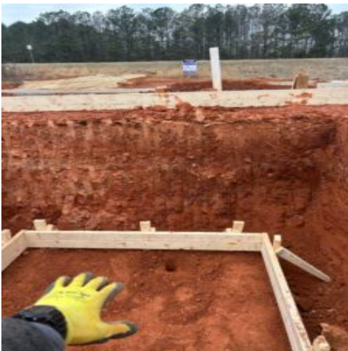
Framing in one of the lift pits.
