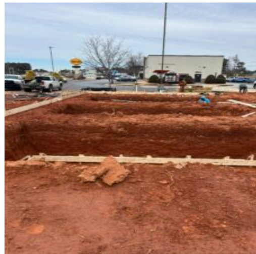
Looking at the lift pits from the south.
