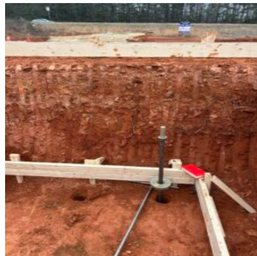
One of the lift pits.
