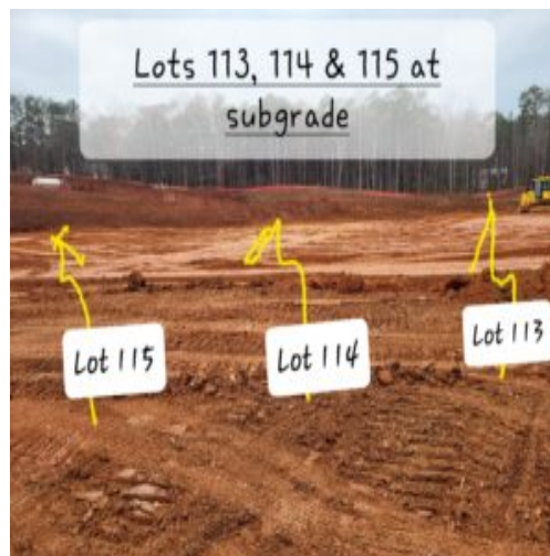
Picture depicting the three building pads at subgrade
