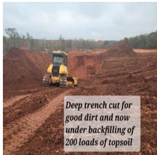
Picture showing deep cut trench under backfilling and packing activity
