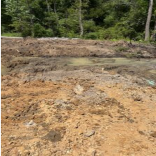
Observed saturated sub grade after excavation
