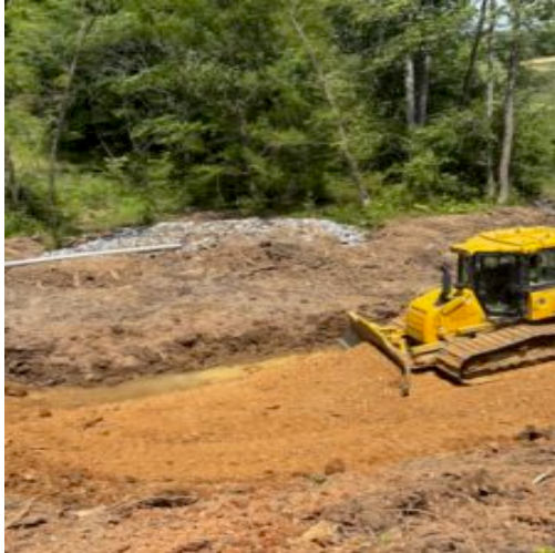
Spreading fill using dozer
