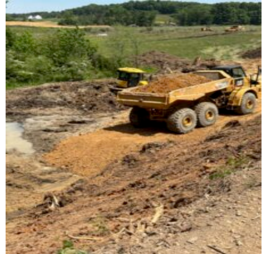
Fill placement using off road dump truck
