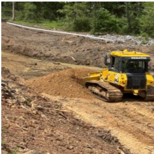
Spreading fill using dozer
