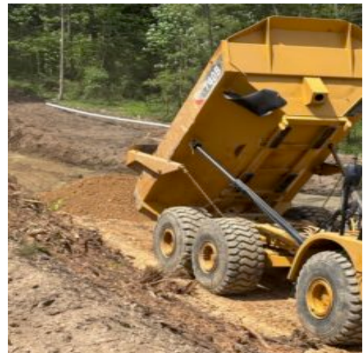
Fill placement using off road dump truck
