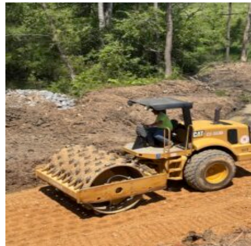
Compacting in place fill using vibratory sheet foot roller
