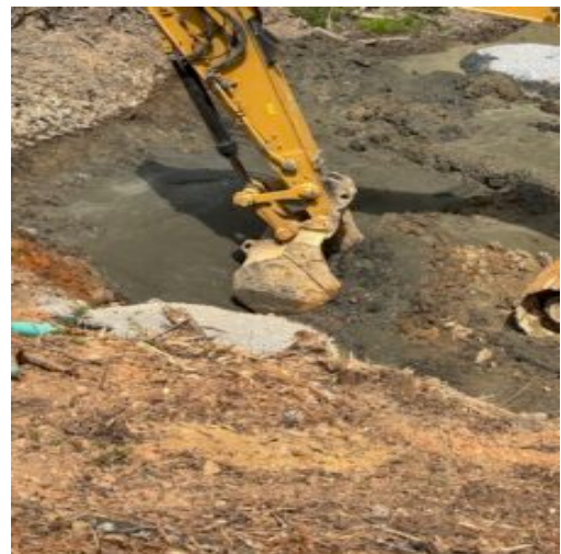
De mucking subgrade prior to placing #57 stone
