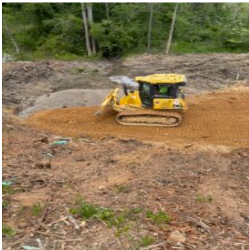
Placing structural fill over #57 stone and filter fabric for subgrade drainage
