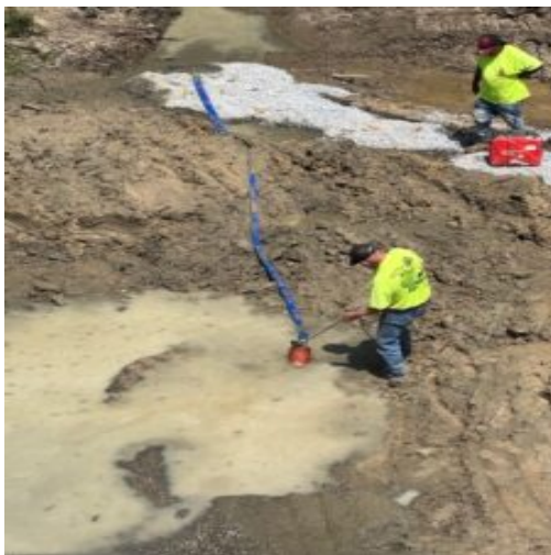
Pumping water prior to placing #57 stone
