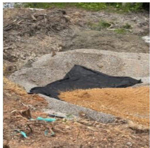
Showing filter fabric over # 57 stone
