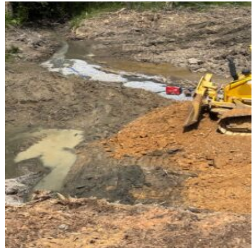
Pushing structural fill over fabric
