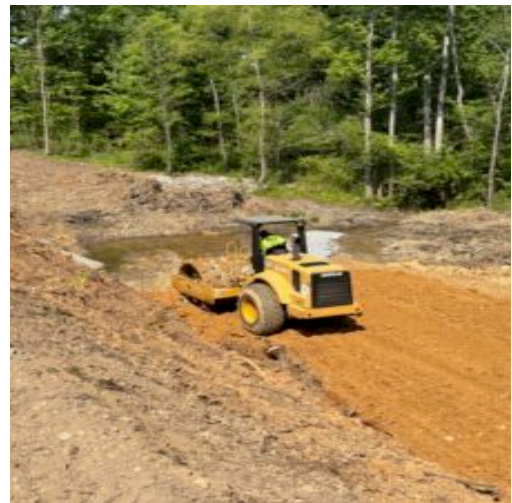
Compacting in place fill using sheet foot roller
