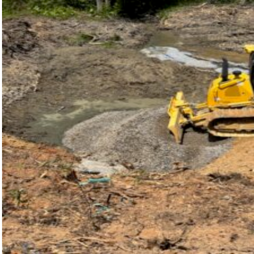
Pushing #57 stone over saturated subgrade for drainage and stabiziation
