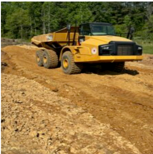
Dumping drier soils
