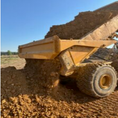
Dumping dry soils for mixing in place
