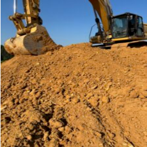
Flipping soils in stockpile for drying
