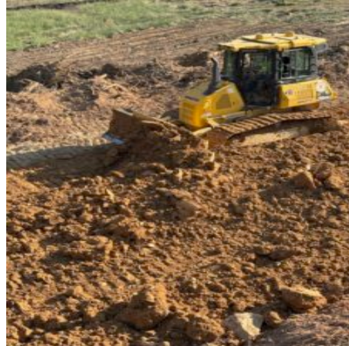
Mixing and plowing dry soils into wet in place soils
