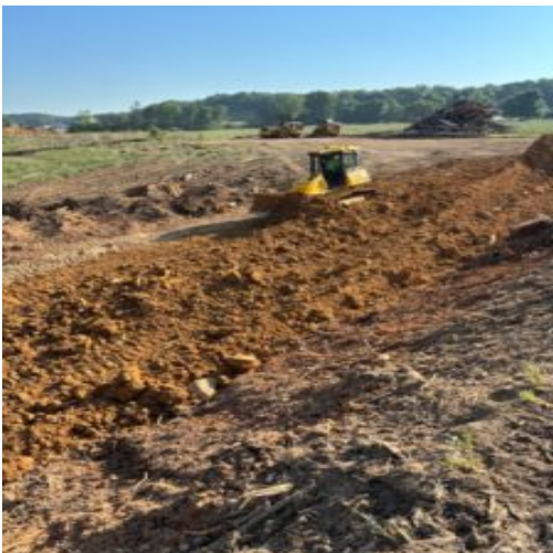
Plowing and blading in place fill soils
