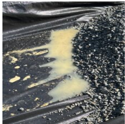
Showing water entering into drain system
