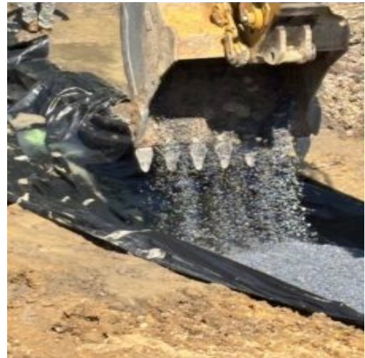
Placing #57 stone onto filter fabric
