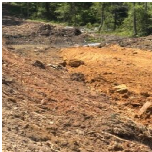
Plowing in place fill placed on 4/21/26 allowing to dry
