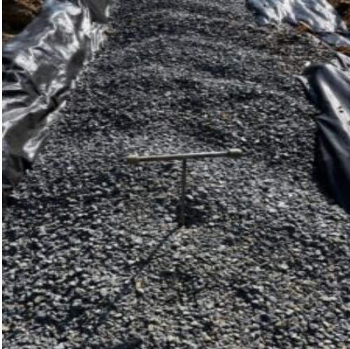
Showing approximately 18" depth of # 57 stone in place
