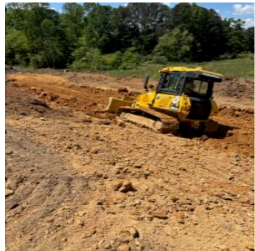
Spreading structure fill over installed drainage system
