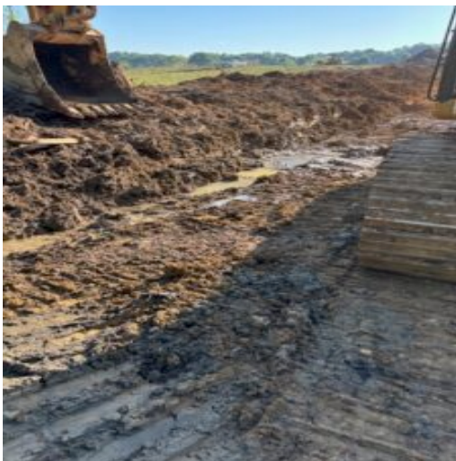
Existing subgrade prior to installing drainage system
