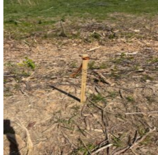
Cut fill stake
