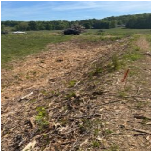
Outside slope embankment looking east with mulch covering
