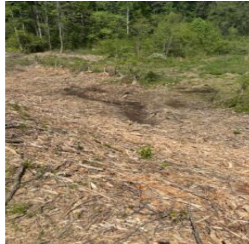
Outside slope embankment looking west with mulch covering
