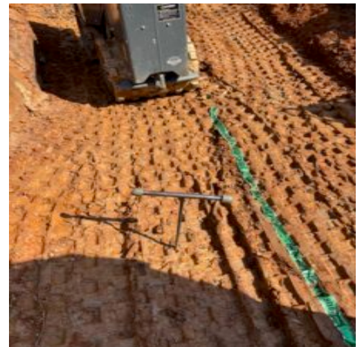
Observed in place fill at sanitary sewer line between ss-2 and ss-1
