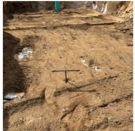
Showing two feet lift prior to blading down
