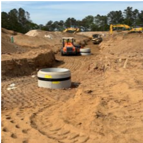
Rock backfill at sanitary sewer line between B12 and B14
