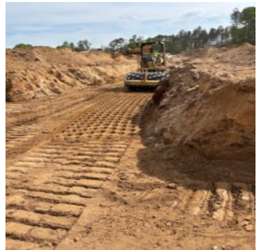
Compacting in place fill
