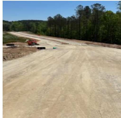
Subgrade prep. at Nature Walk Pkwy. between manhole # 10 and 11
