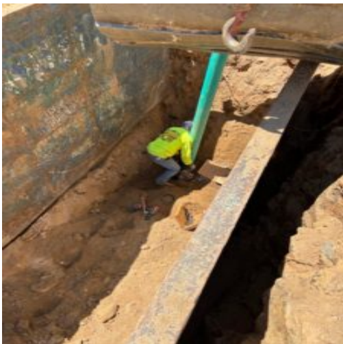
8" ductile iron sanitary sewer line and laterals between B13 and B14
