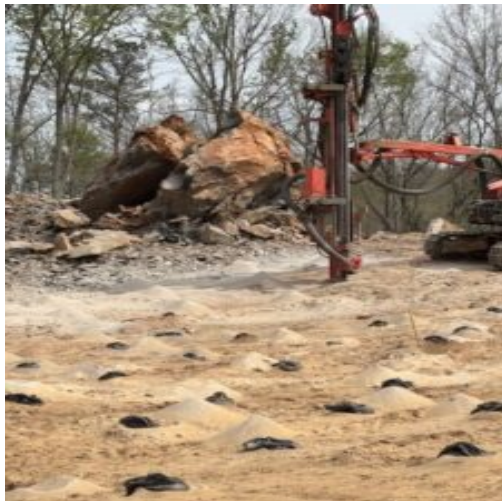
Drilling at cul de sac
