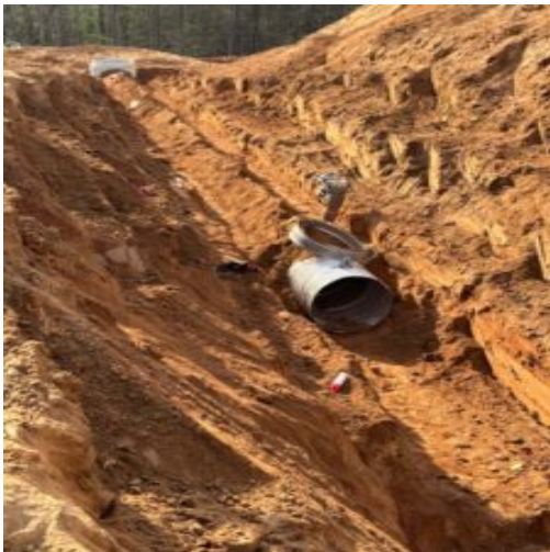
Installing 36"cmp storm line between A6 and A7
