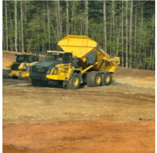
Hauling blast rock
