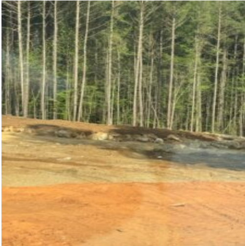
Placed blast rock at unit 4 phase 3
