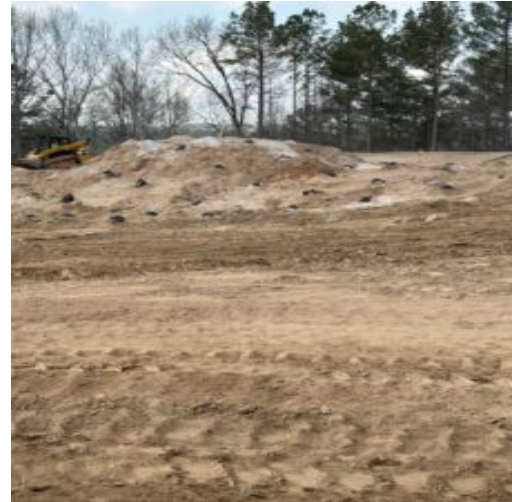
Drilled at lot # 37
