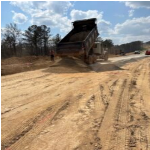
Sub grade prep. dumping base stone
