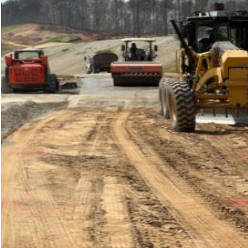
Compacting in place contract base stone
