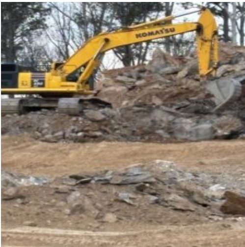
Moving blast rock from blast lots
