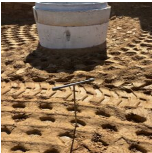
Backfill observation probe testing.
