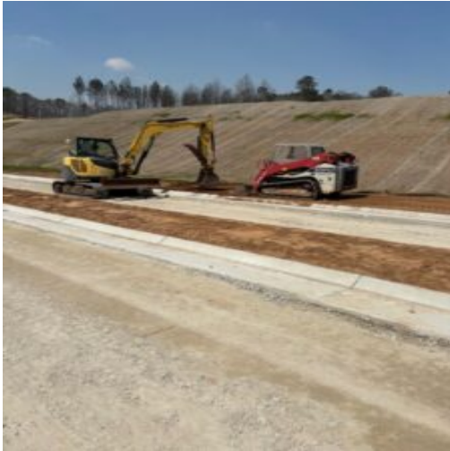
Grading contractor backfilling curb
