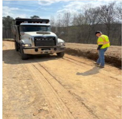
Proof rolling sub grades
