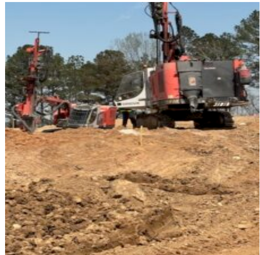
Drill rigs at lot #37
