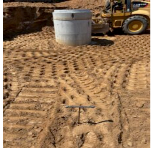
Back fill observation and probe testing
