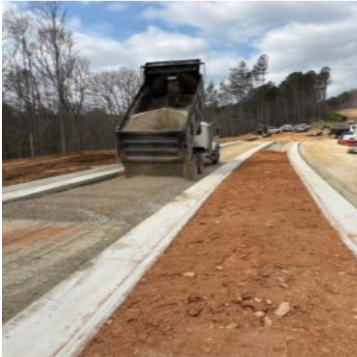
Adding additional base stone at repair areas
