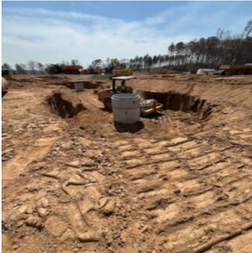
Backfill and compacting r.c.p. 30" storm line
