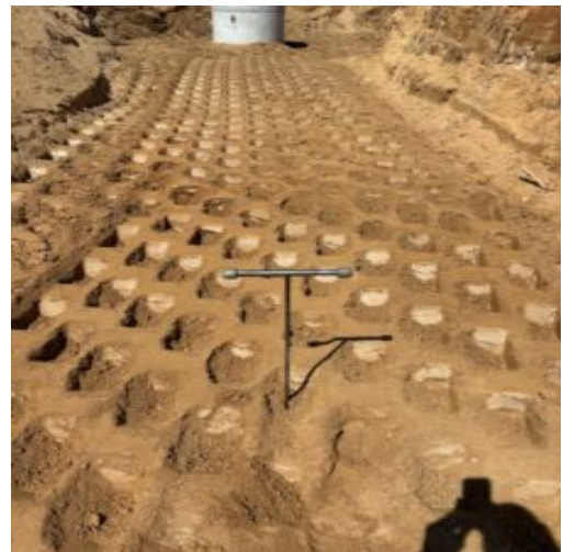
Backfill observation probe testing
