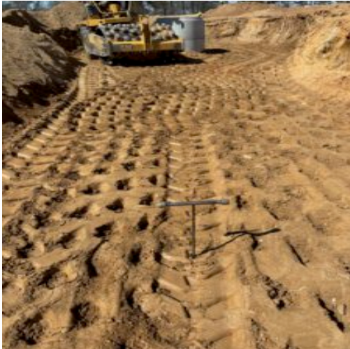
Backfill observations probe testing recommended additional testing
