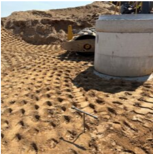
Backfill observations and probe testing recommended for additional compacting
