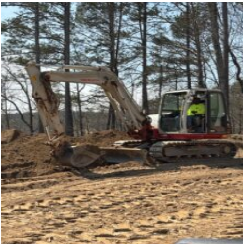
Water line contractor installing 8" water d.i.p. line
