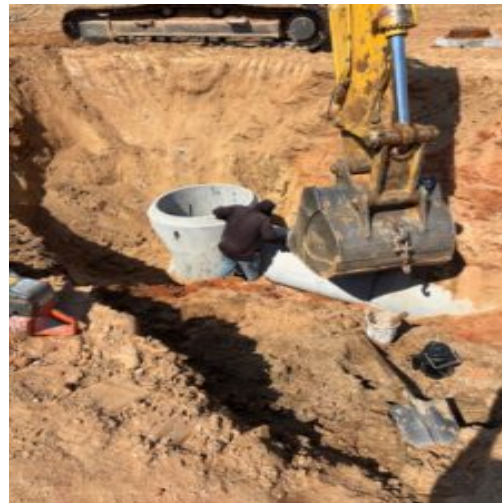
Installation of 30" rcp storm and backfill between B5 and B6.
