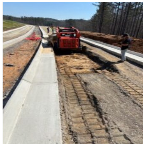
Sub grade repair at Nature Walk
