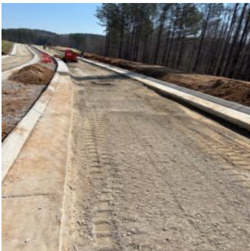
Sub grade repair at Nature Walk
