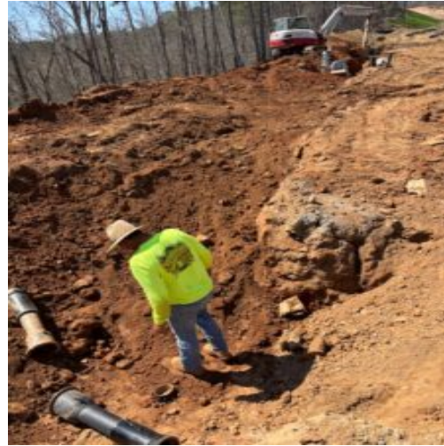
Water line installation and backfill at Nature Walk
