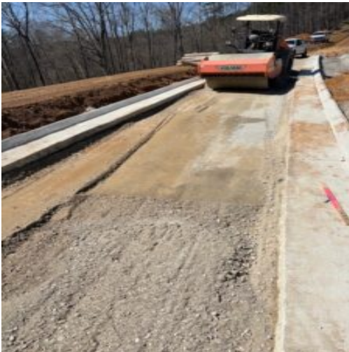
Subbase undercut and repair at Nature Walk pway.
