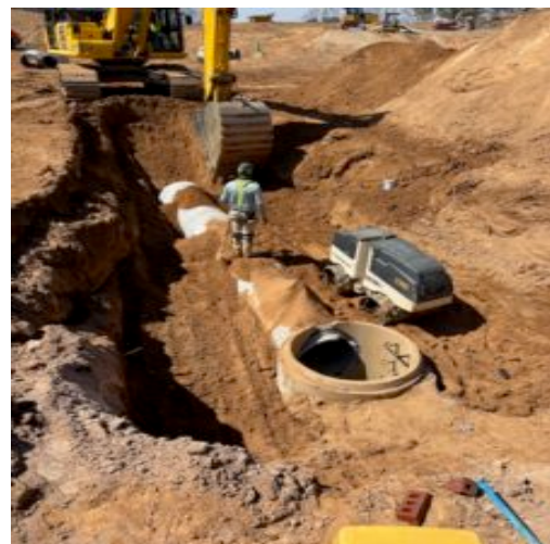
Installation and backfill at 30 " rcp storm line between B4 and B6
