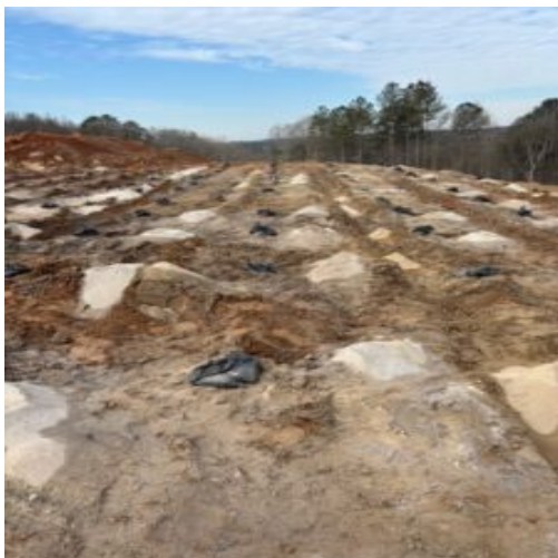
Drilling preparing for blast
