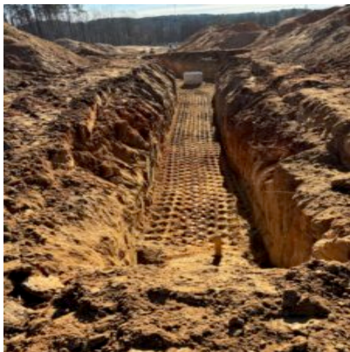
Sanitary sewer trench backfill between B9 and B10
