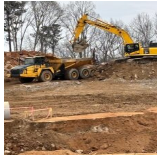
Loading rockfill from blast area
