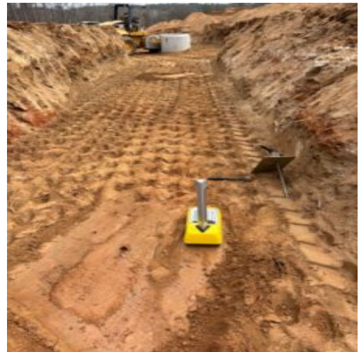
Performing density tests between B9 and B11
