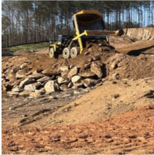
Dumping rockfill at slope embankment green area
