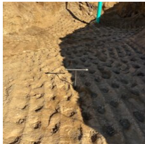
Probing to request additional compacting
