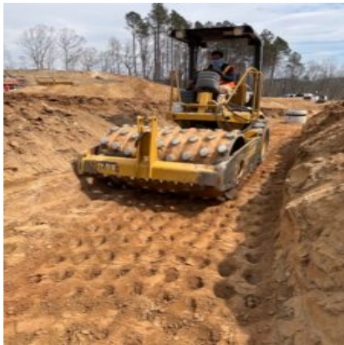
Compacting fill between B9 and B11
