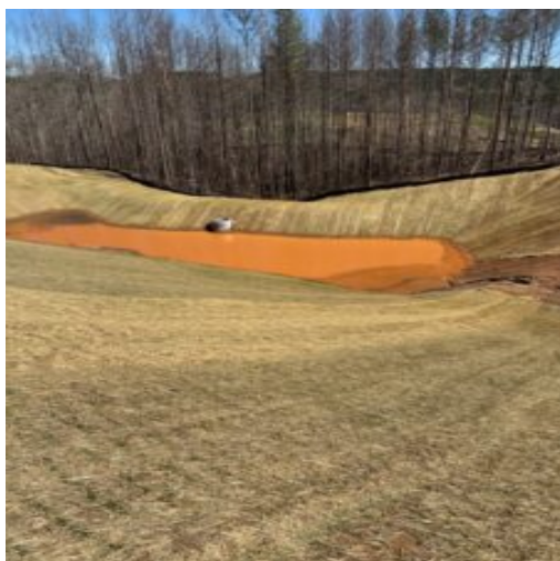
Detention pond after rain event
