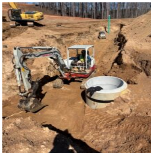
Backfill and compacting efforts at sanitary sewer trench
