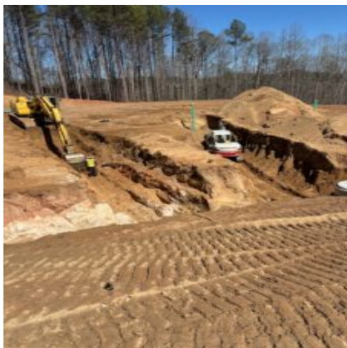
Installing lateral clean outs and backfill
