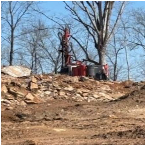
Drill rigs drilling
