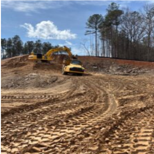
Fill placement at lots # 33 thru 36 and density tests performed
