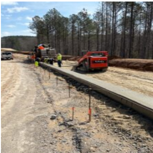
Curbing (1500) feet poured at Nature Walk boulevard.
