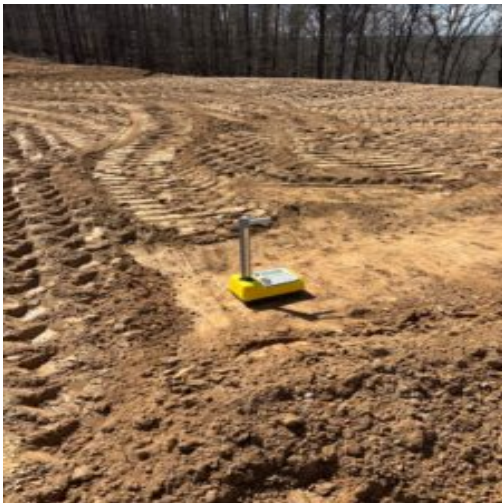
Fill placement at lots # 33 thru 36 and density tests performed
