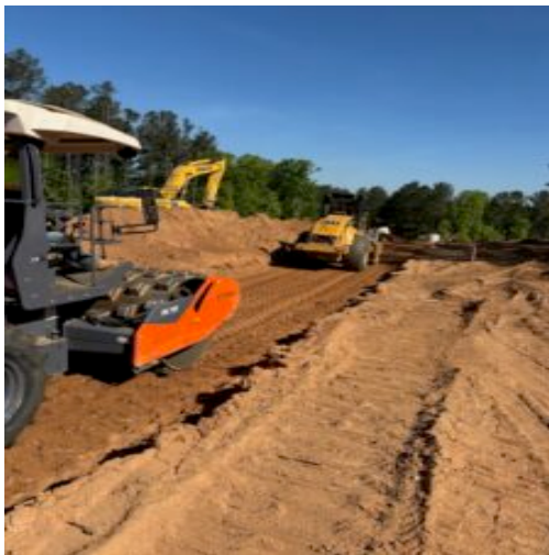
Compacting in place fill using two sheet foot rollers.
