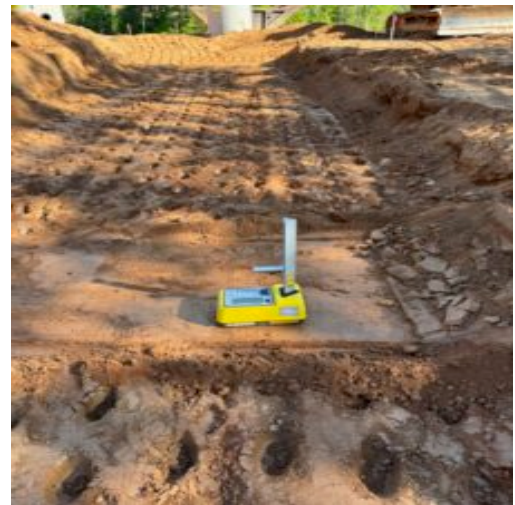
Performing density tests using Nuclear Gauge
