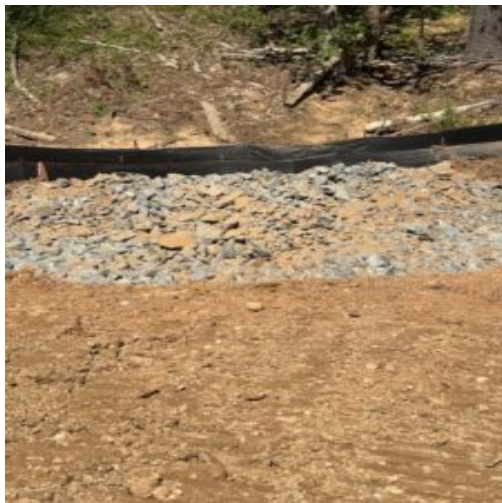
Rip Rap place at OCS headwall structure
