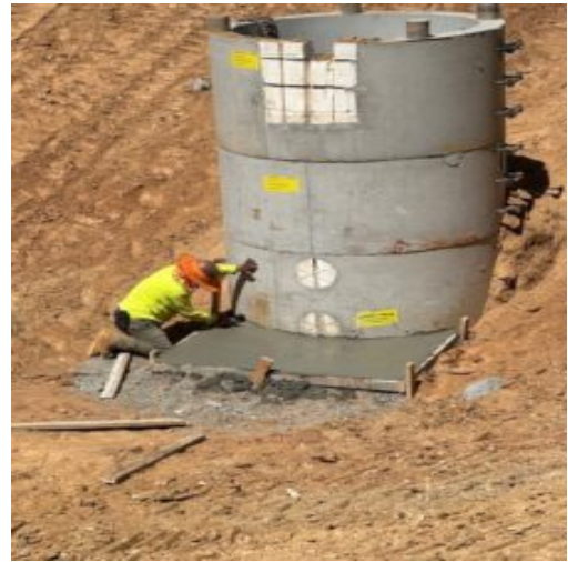
Pouring concrete base for trash rack
