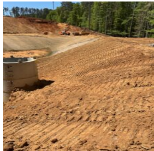
Completed backfill at dam embankment
