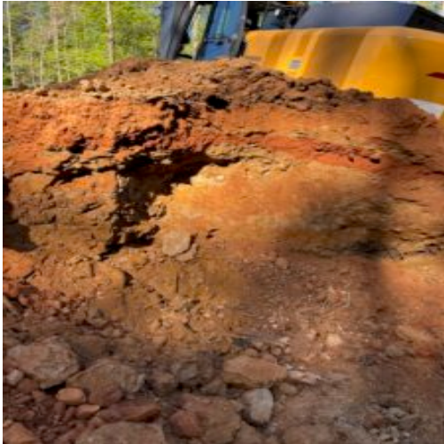
Excavated organic fill replaced with suitable dry materials
