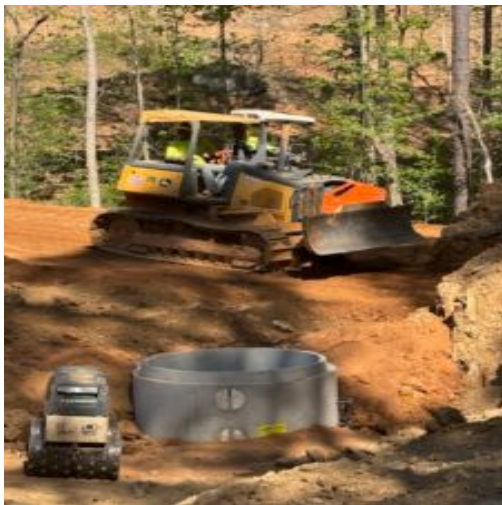
Fill placement and compacting efforts
