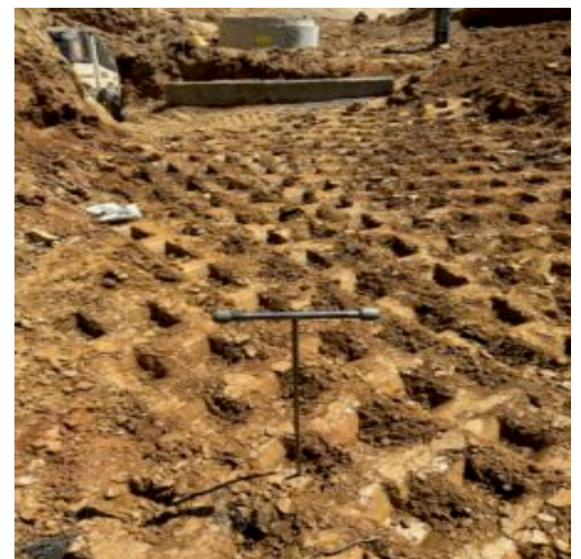
Backfill placement and observation by using a probe rod for testing which compacting efforts were suitable for requirements.
