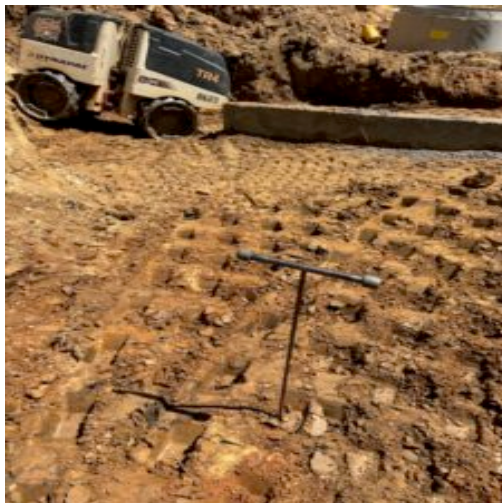
Backfill placement and observation by using a probe rod for testing which compacting efforts were suitable for requirements.
