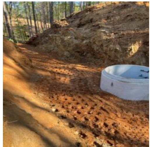
Backfill at OCS storm line
