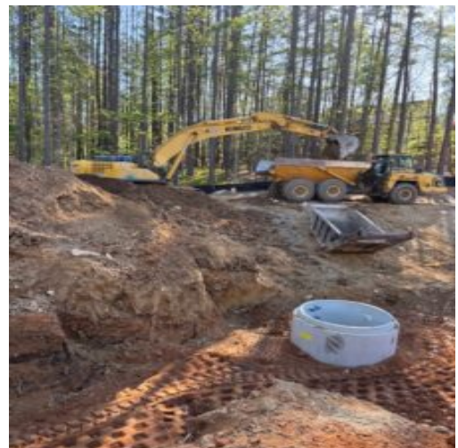
Backfill at OCS storm line
