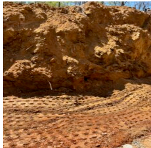
Compacting using walk behind vibratory sheet foot roller
