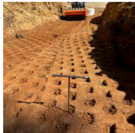
Probing suitable for compaction requirements
