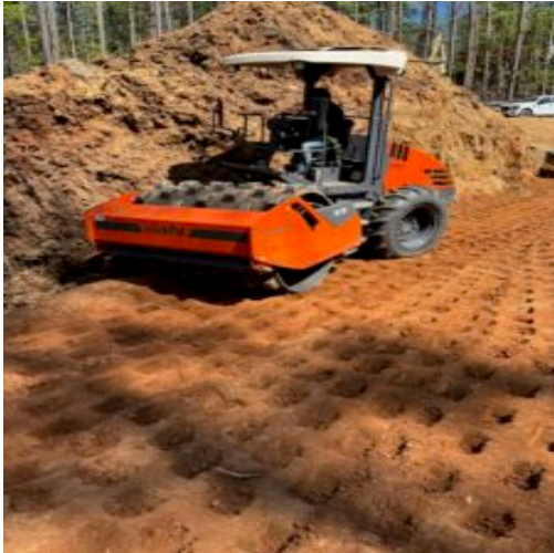
Compacting using vibratory sheet foot roller
