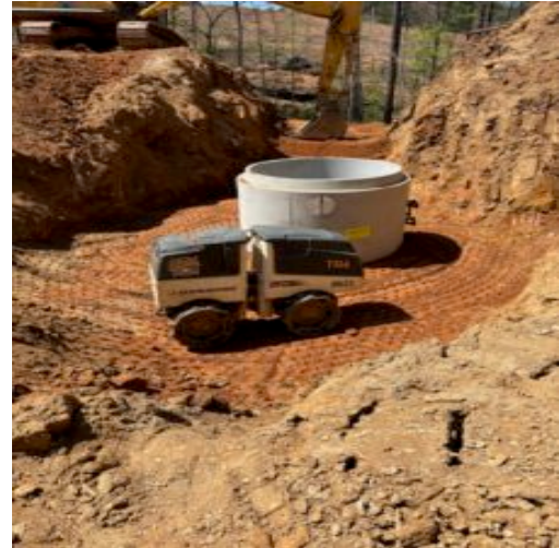
Compacting using walk behind vibratory sheet foot roller
