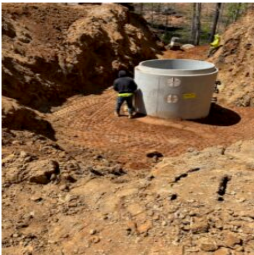
compacting using hand tamp
