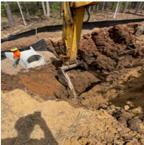
Excavating unsuitable materials at back of slope embankment
