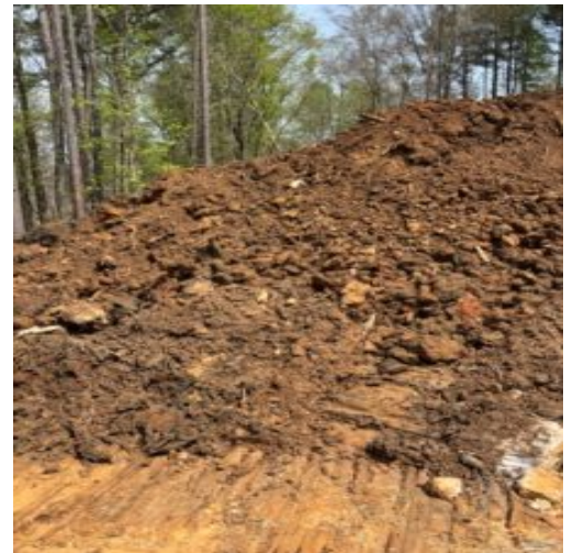
Excavating unsuitable materials at back of slope embankment
