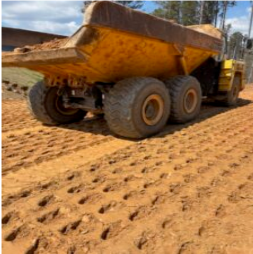
Compaction efforts observed by proof rolling and probing.
