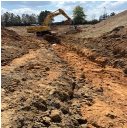
Installation and backfill of 30" cmp storm line
