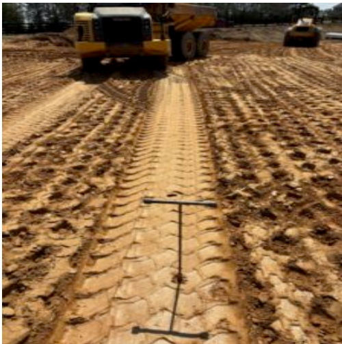
Compaction efforts observed by proof rolling and probing.
