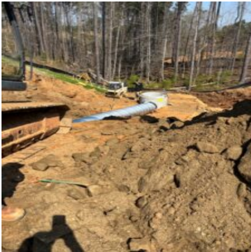
Installation of 30" cmp storm line between G2 and G3
