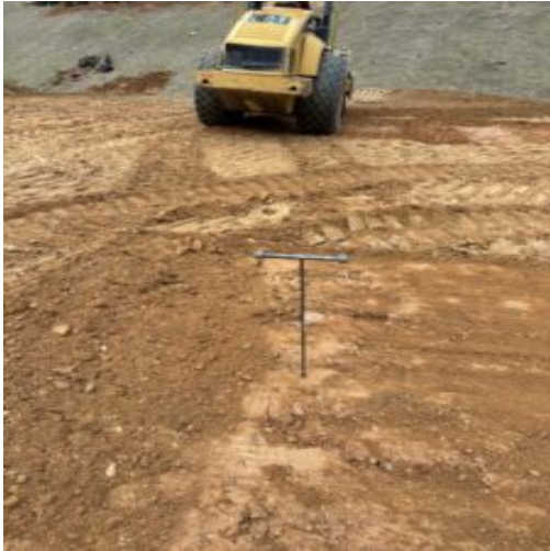
AM probing in place fill suitable for compaction at -7'
