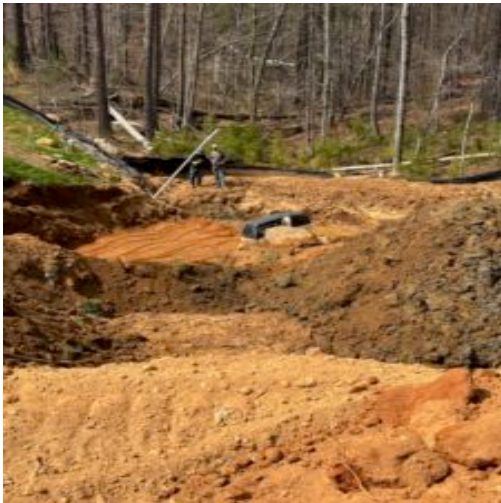
AM probing in place fill suitable for compaction at -7'
