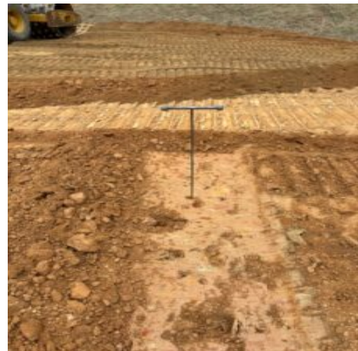
AM probing in place fill suitable for 95% compaction at -7'
