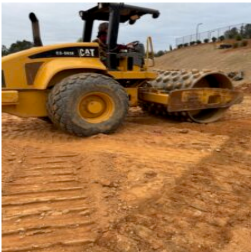
Compacting efforts at elevation -7'
