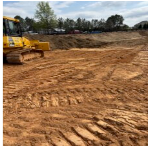
Fill placement at old detention pond
