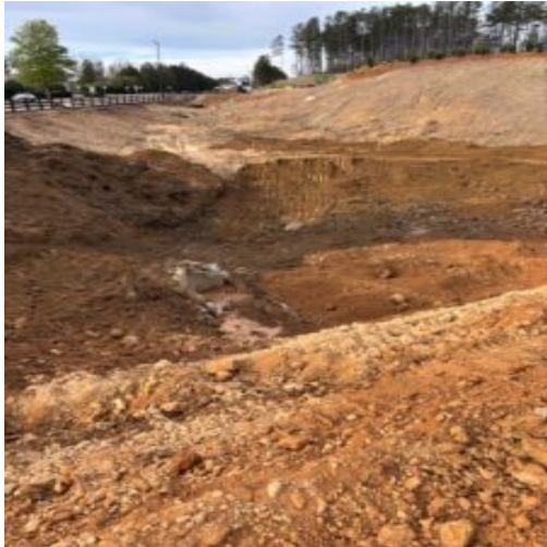
Excavation demucking at old detention pond
