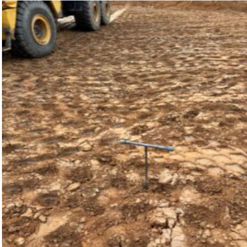
Probing in place fill
