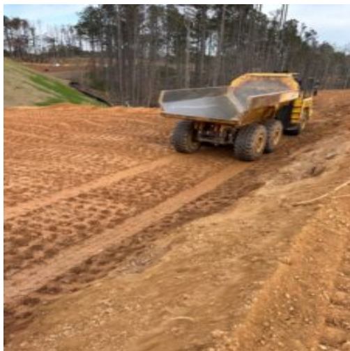
Proof roll compacting efforts
