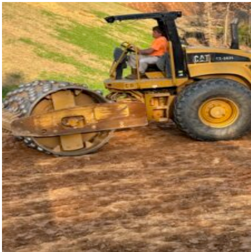
Compacting in place fill
