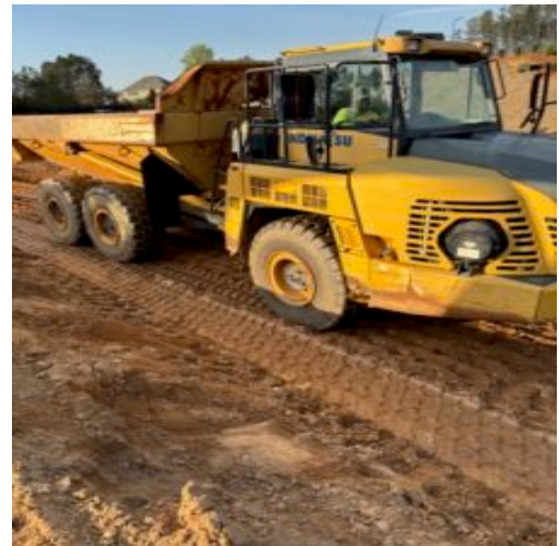
Observing in place fill by proof rolling
