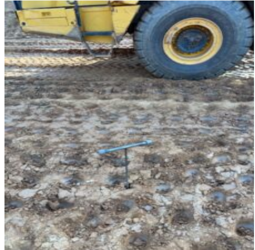
Probing in place fill using rounded end steel rod
