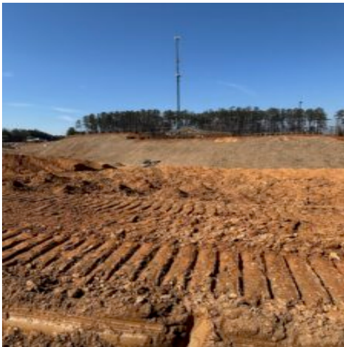
Observing in place plowed soils for drying at lots 41 and 42
