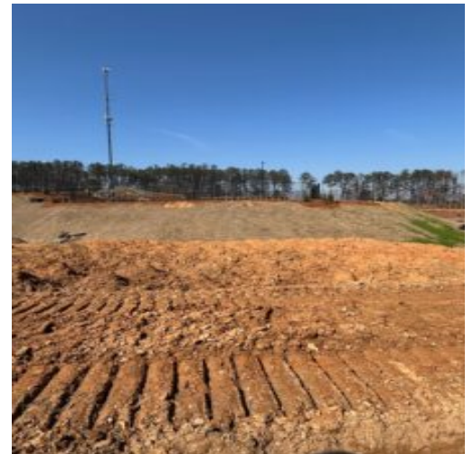
Observing in place plowed soils for drying at lots 41 and 42
