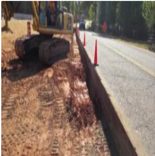
decel lane remediation
