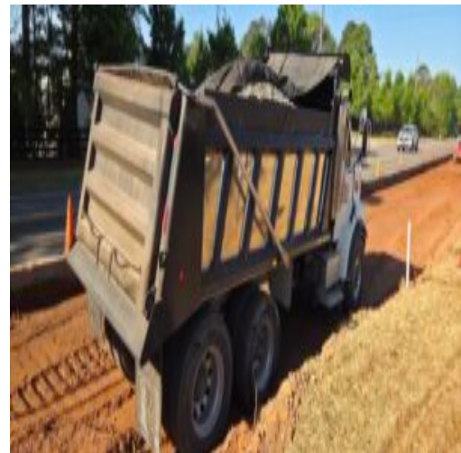
loaded truck for proof roll
