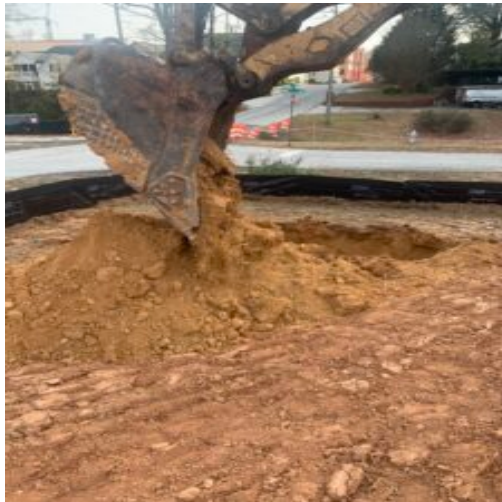
Obtaining proctor samples #2 and 3 at SW corner of site
