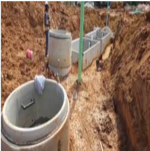
grease traps in middle of the site
