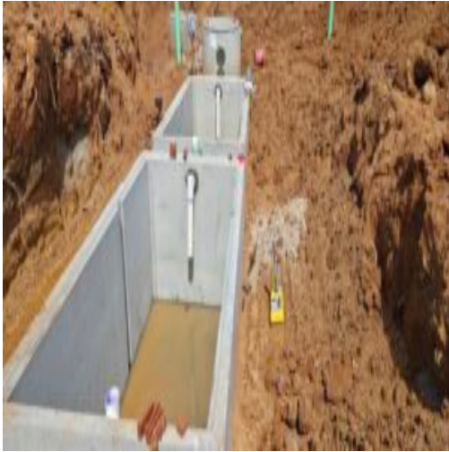
grease traps in middle of the site
