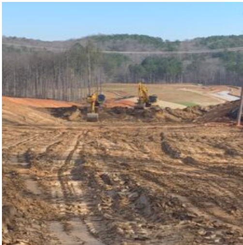
Undercutting rock fill from Nature Walk Parkway near sanitary sewer manhole #9
