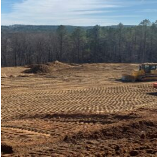
Fill placement at slope embankment
