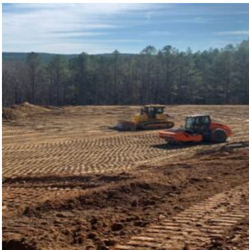
Fill placement at slope embankment
