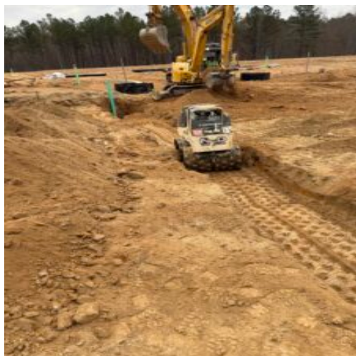
Backfilling over pipe
