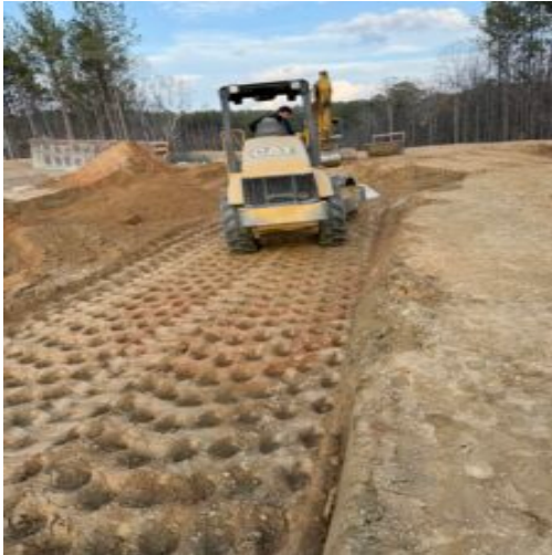
Trench compacting
