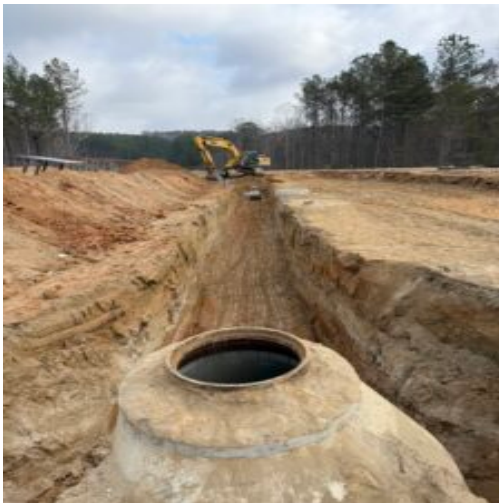
Trench area backfilling
