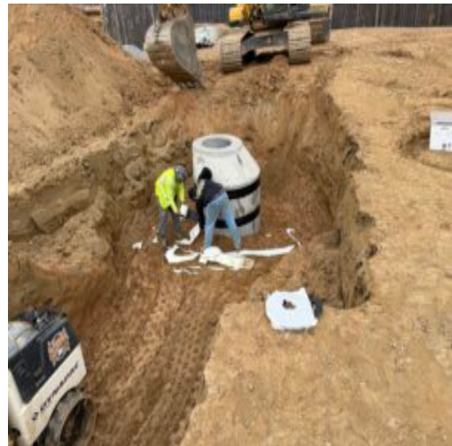
sealing manhole trench area
