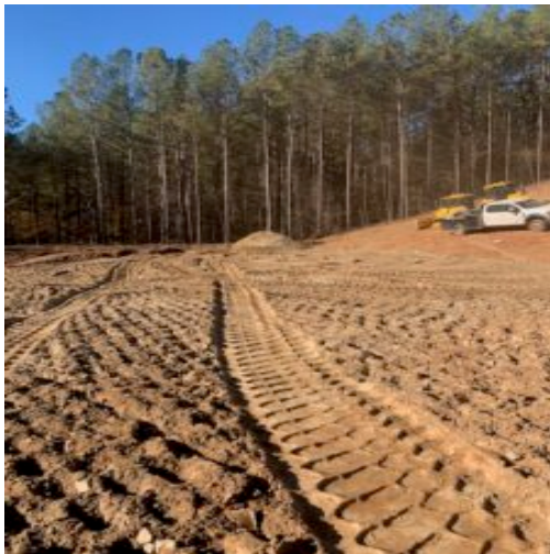
Rock fill placement at slope embankment
