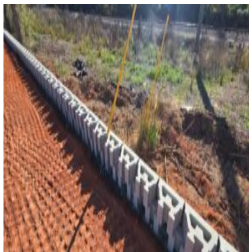
wall splits support wires for telephone pole
