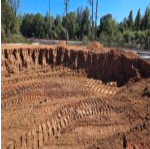
roadway bench cut out of slope on retaining wall
