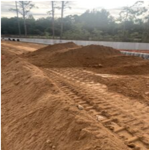
Fill placement at wall
