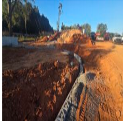
retaining wall and fill already on site
