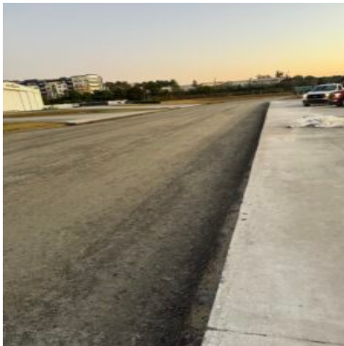
Alpha ramp with recycled concrete placed
