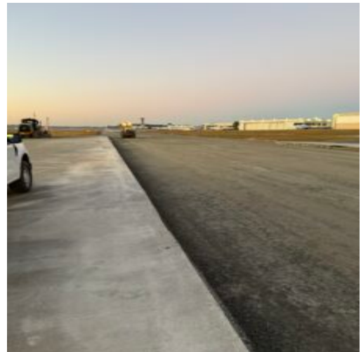
Alpha ramp with recycled concrete placed
