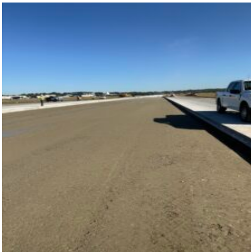
Runway Keel with recycled concrete
