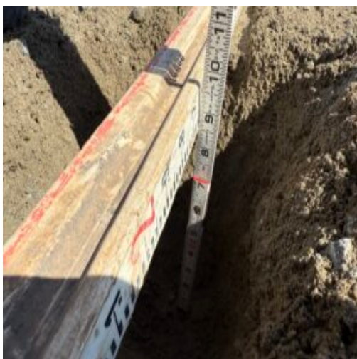
Checking Recycled concrete depth
