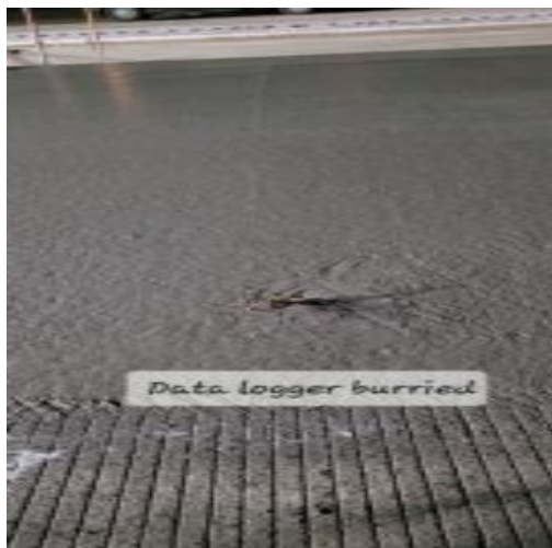
Data logger inserted at the concrete for future temperature monitoring
