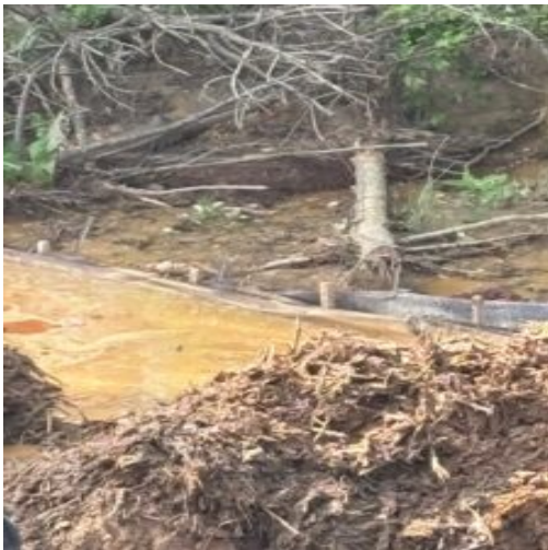
Deficient area due to rain event at toe of slope
