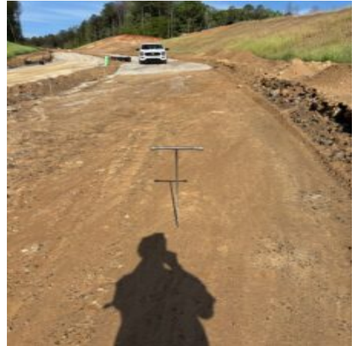
Sub grade approved for base stone placement
