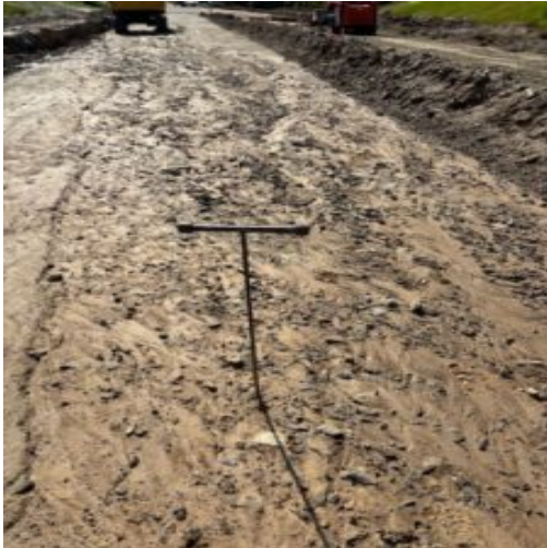
Washed sub grade area approved for stone placement
