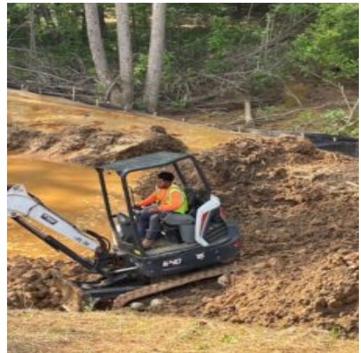
Repairing deficient area at toe of slope
