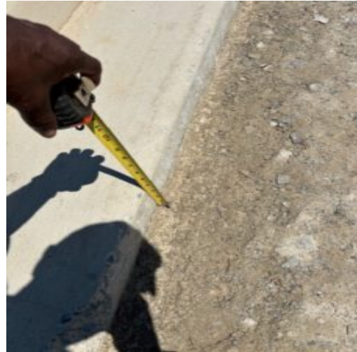
Subbase prep.at Nature Walk Pkwy. showing sufficient depth for asphalt.
