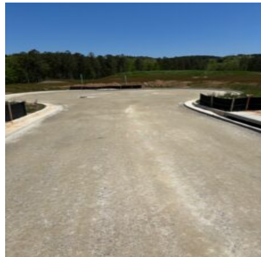
Subbase prep.at phase 1A
