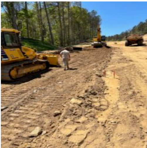
Subgrade prep.at Nature Walk Pkwy. undercutting 8" to 12"
