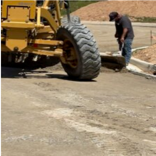
Subbase prep.fine grading at Nature Walk Pkwy.
