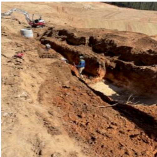
24" cmp storm line installation at C line
