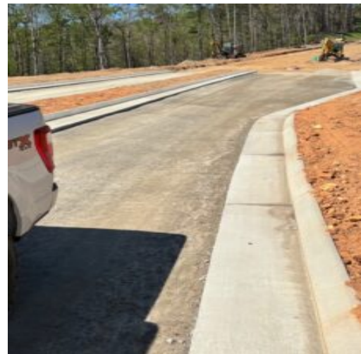
Subbase prep. at Nature Walk Pkwy.
