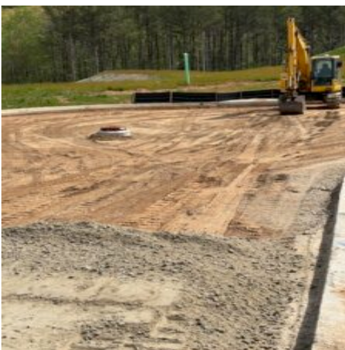
Subgrade prep. at cul de sac
