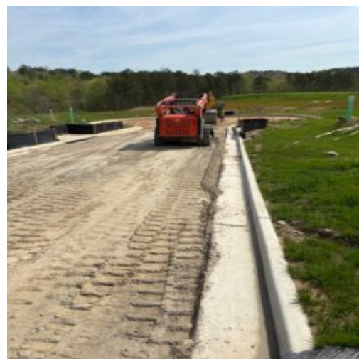
Subbase prep. compacting in place base stone
