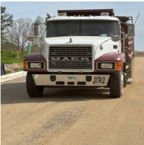
Observing test proof roll of subbase
